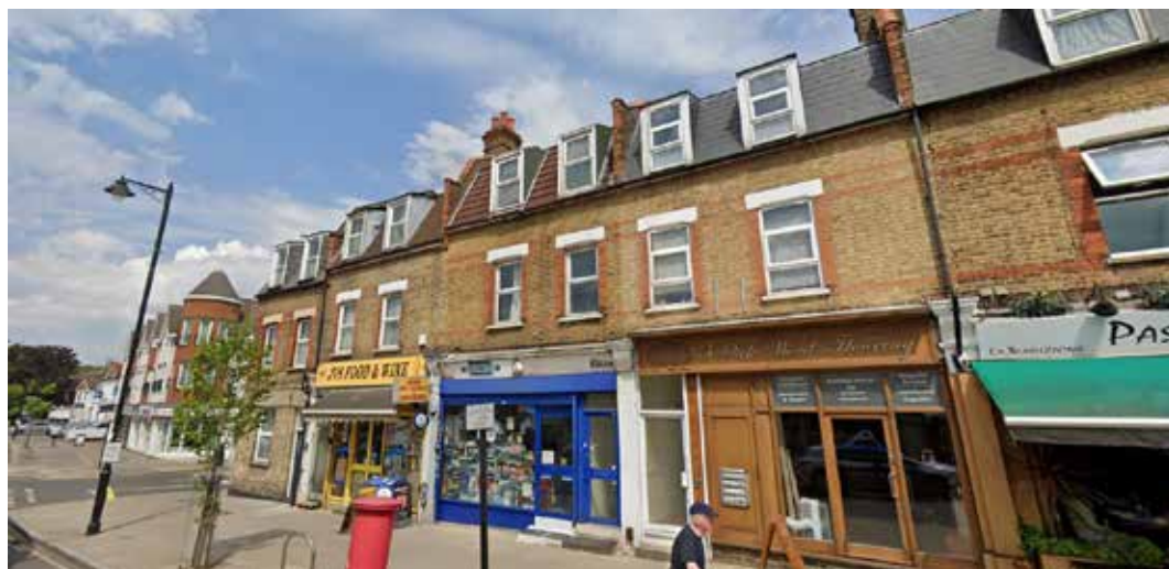
No's. 213-221 Northfield Avenue (3-storey with mansard roofs)
