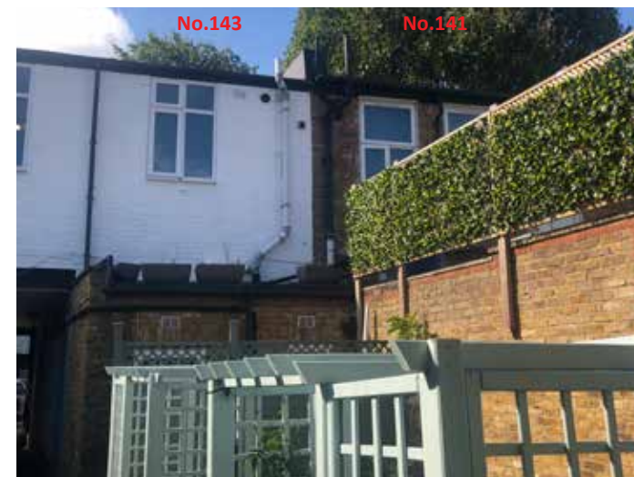
Rear elevation of nos. 141-143 Northfield Avenue (east facing)
