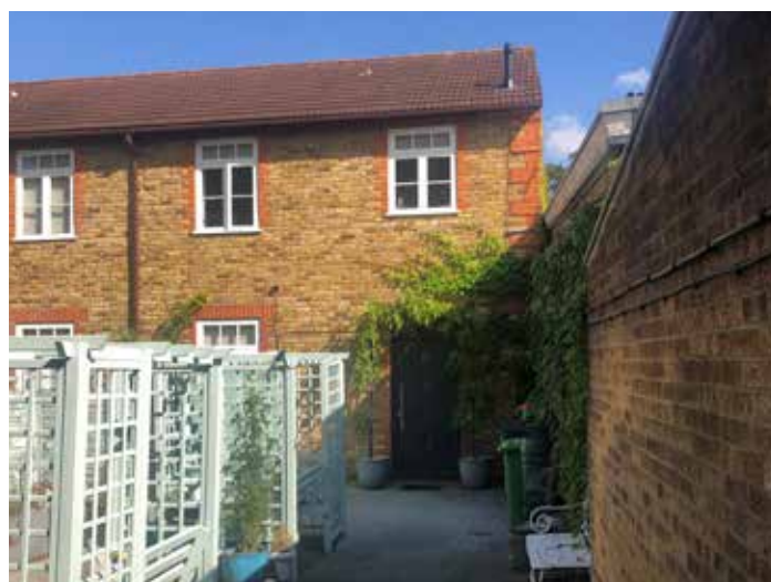
Rear building at no.143 Northfield Avenue (west facing)
