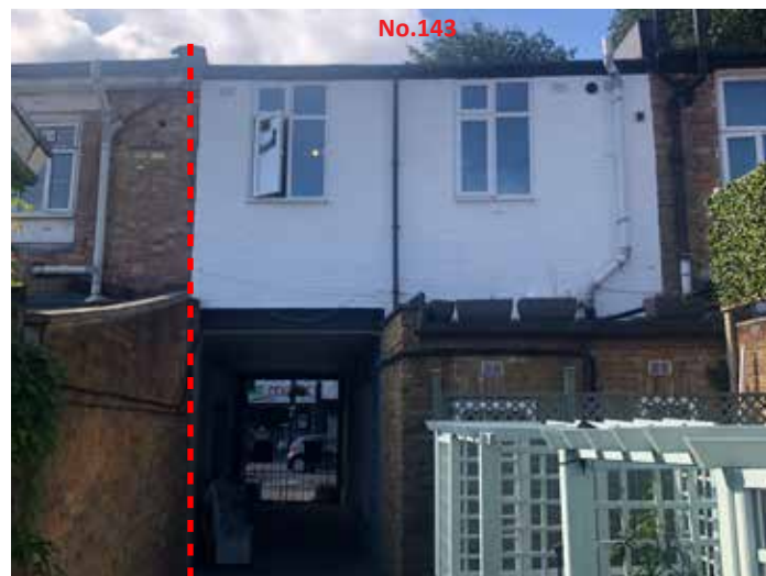
Rear elevation of no. 143 Northfield Avenue (east facing)
