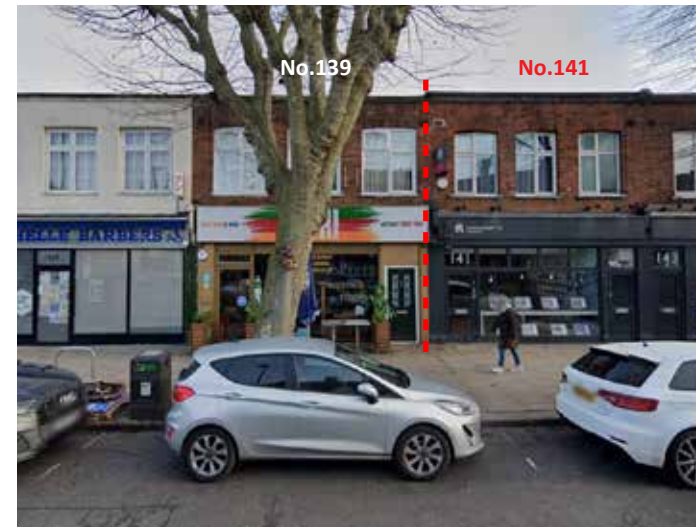
Neighbouring buildings nos.137-139 Northfield Avenue
