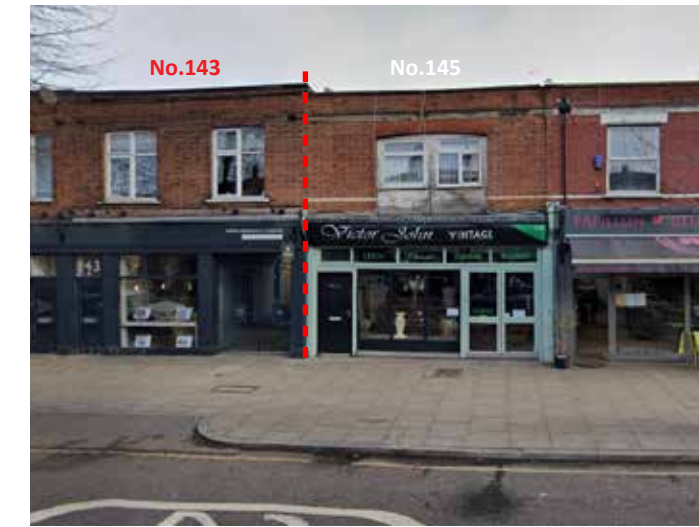
Neighbouring buildings nos.145-147 Northfield Avenue
