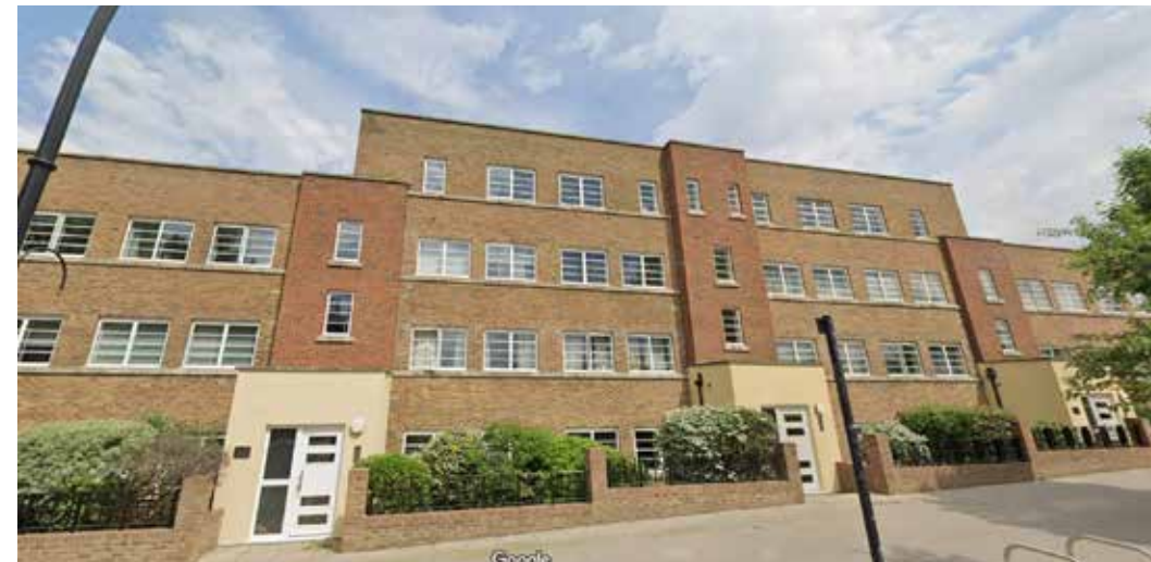
No's. 1-30 Derwent Yard (3-storey with flat roofs)
